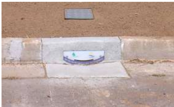
Photograph 4. and Figure 10. Salisbury Council behind the kerb design using the TREENET inlet faceplate
