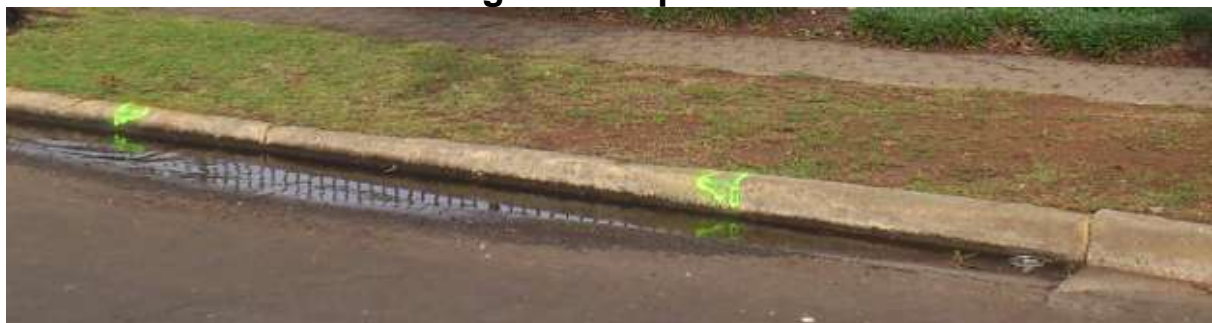
Photograph 3. Vertical kerb lift resulting in ponding
